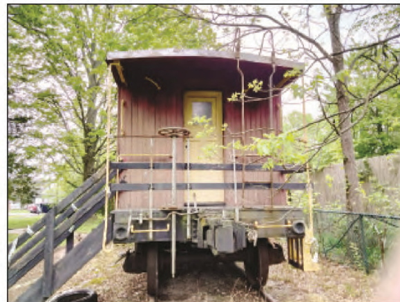
Another view shows the deteriorating caboose.
